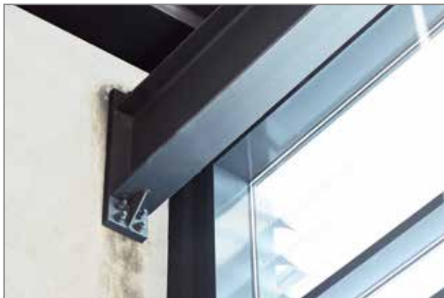
Figure 11: Thermal bridging occurring at continuous steel beams.
