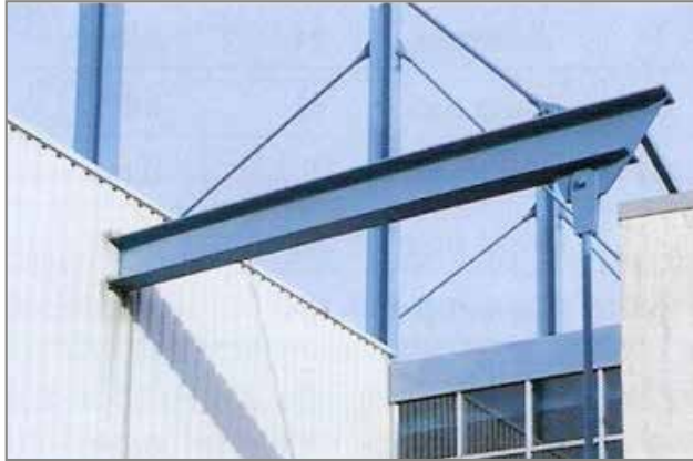
Figure 10: Structural thermal bridging in steel structures.
