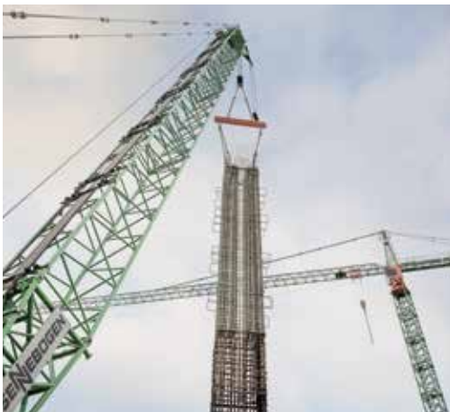
2nd S-Bahn trunk line, Munich (©Moritz Bernouilly)
