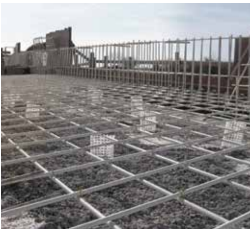
Reinforcement of the bridge coping at Canal Bridge, Canada
