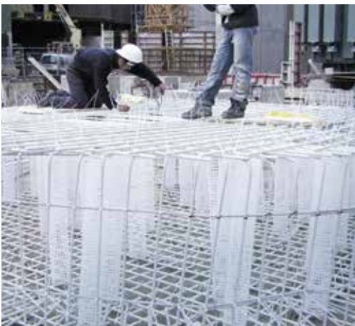
Foundation reinforcement in the transformer house of Peiner Träger GmbH, Peine
