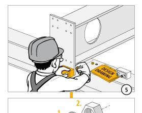
(5) Install Schöck Isokorb® Type S22 according to the design drawings on the head plate of the steel beam within the building shell.
